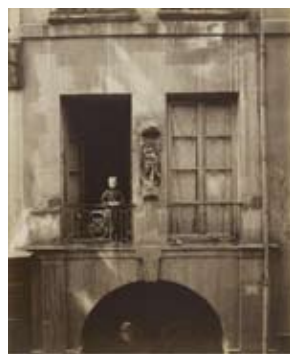
The former College de Chanac, 12 rue de Bievre, 5th arrondissement August 1900 Albumen photograph @ Musee Carnavalet, Paris/ Roger-Viollet/ TopFoto
